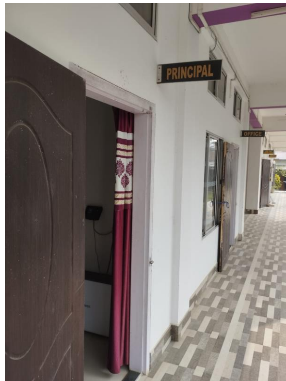
Principal's Room (Outside)
