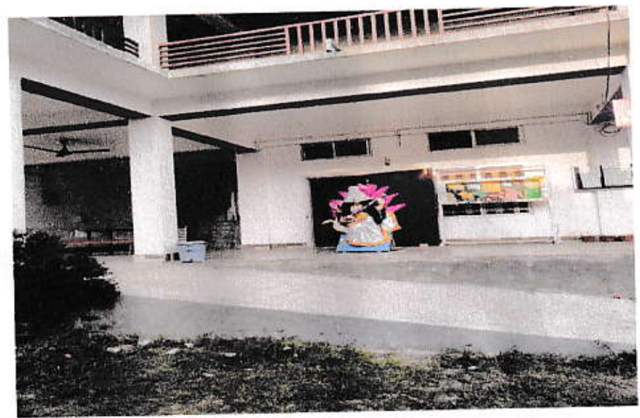
Ramp (Entrance Gate)
